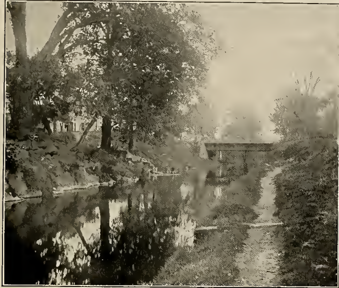
The Boulevard Bridge over the Morris Canal
